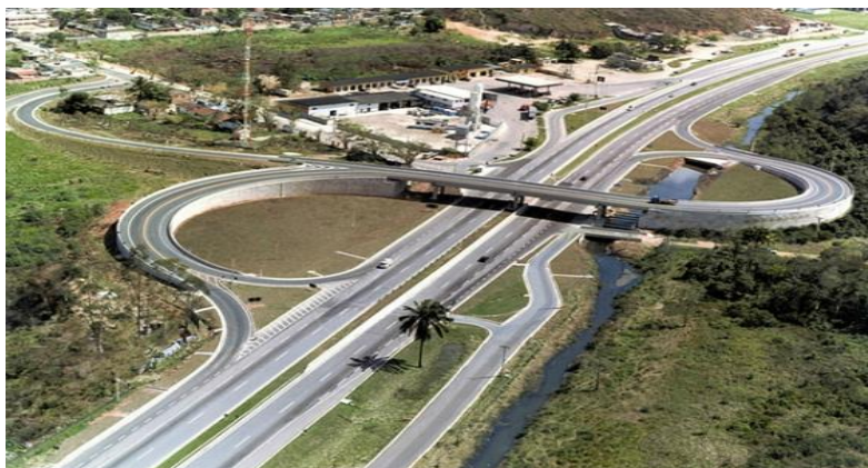
Figure 1. Images of the highway infrastructure of the company. Source: CRT (2018a).
